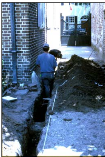
Figure 26: excavation of the service trench
