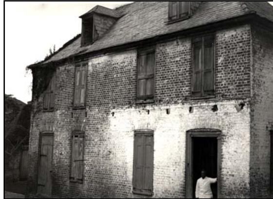
Figure 15: the kitchen building with whitewashed first floor exterior.
